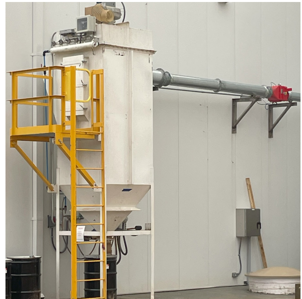
The Dust Collector is sized to meet the total demand of the system provided, plus a safety factor. Complete feedback of the entire DC system ensures reliability. XP features are provided including Isolation Valves and Rupture Panels or Flameless Vents.
