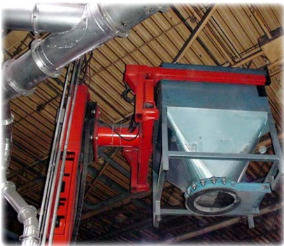
IBC being set in place by Column Lift
