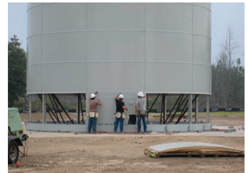
Standpipe - jacked from grade level
