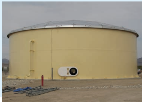
Field-weld - Potable water
