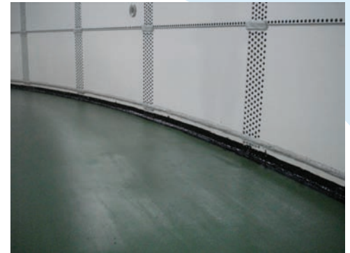
XL Municipal Water Storage Interior Base Setting Ring with Concrete Bottom
