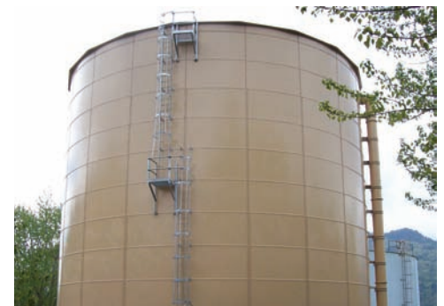
RTP Construction - Potable Water
