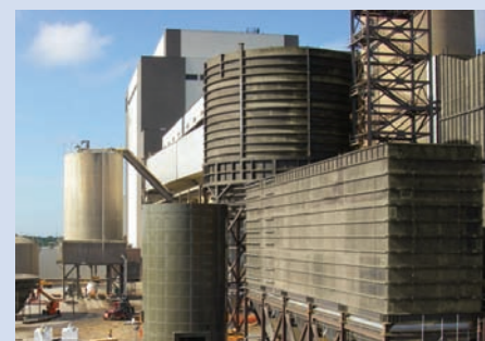
Bolted RTP, Field-weld & Hybrid Tank Construction
