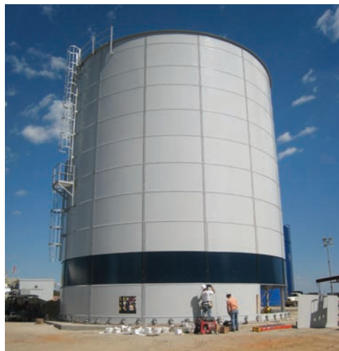
Power Utility - Process Water
